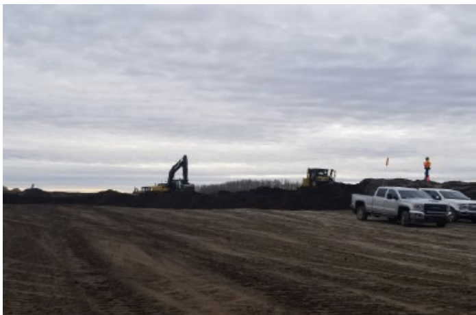
Topsoil replacement on ROW – SF 31 – Oct 15, 2018
