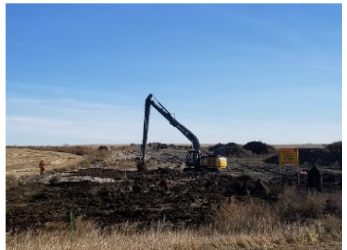
Long stick working to dry out soils – SF 44 - Oct 19, 2018
