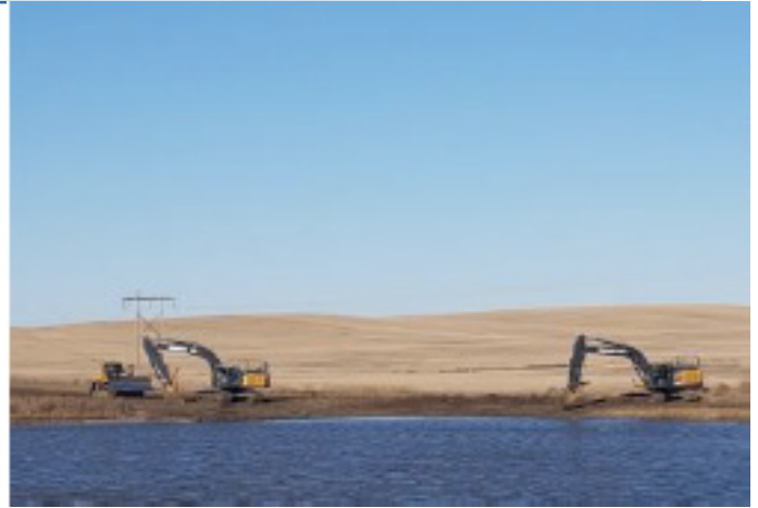
Wetland ramp removal – SF 41 - Oct 21, 2018
