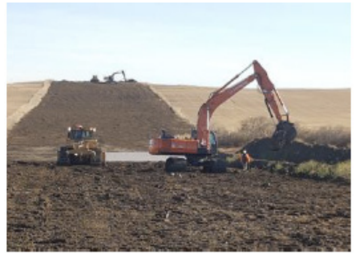
Working on wetland – SF 41 - Oct 19, 2018
