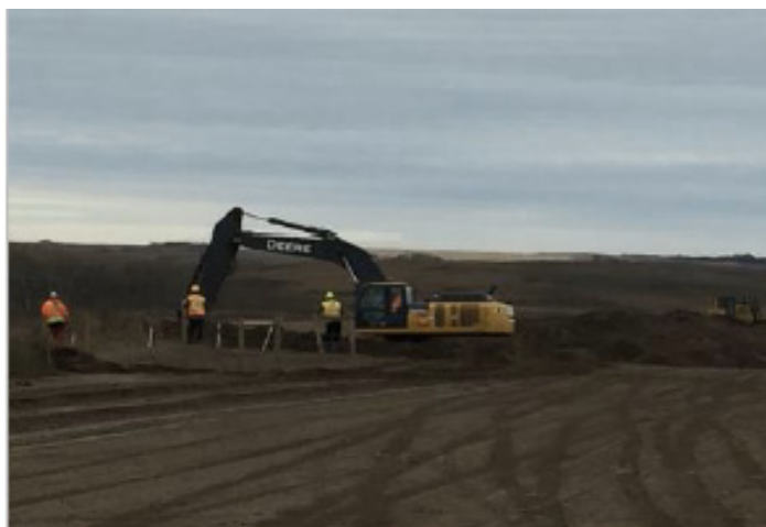
Excavator pulling topsoil – SF 60 – Oct 15, 2018
