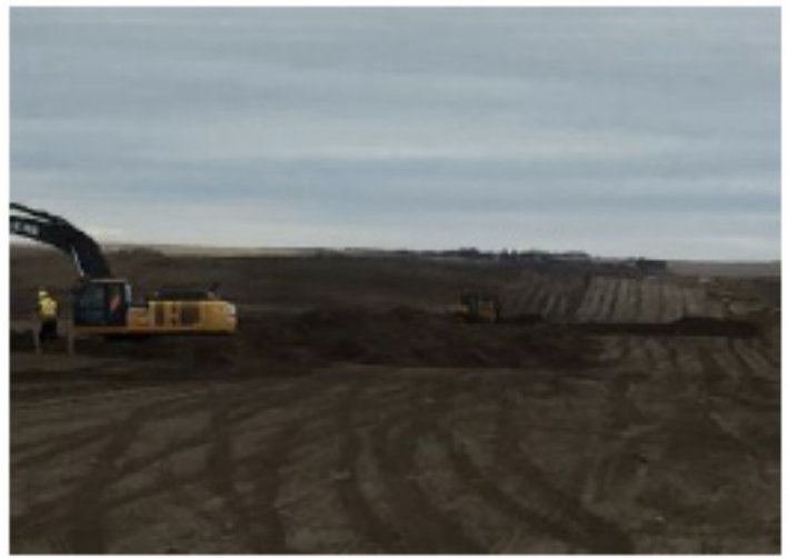
Excavator and dozer pulling top soil on ROW– km 99+900 - Oct 15, 2018
