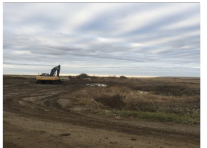
Ramp removal – SF 30 – Oct 16, 2018
