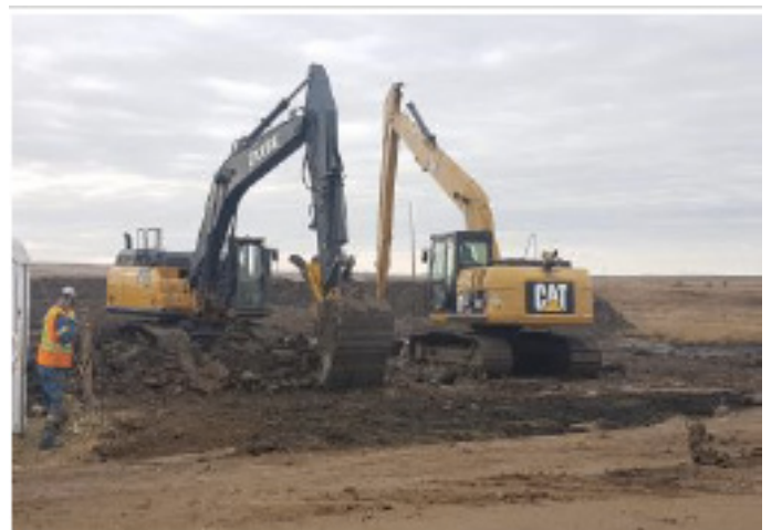
Excavator working on ramp removal – SF 39 – Oct 16, 2018
