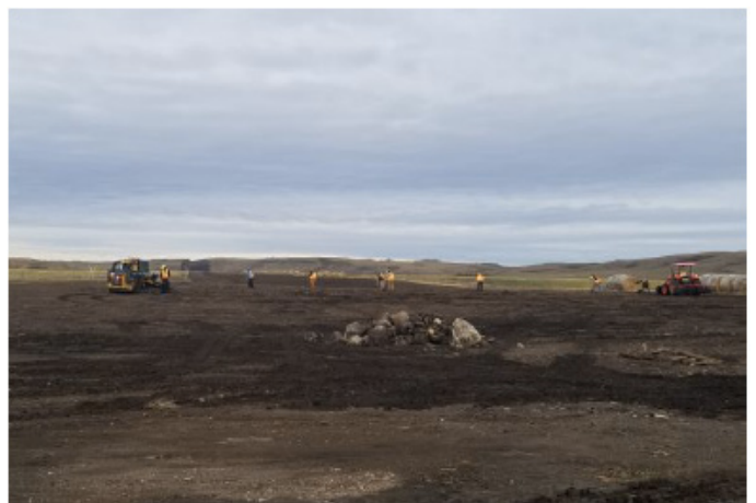
Rock picking and piling on ROW – SF 28 - Oct 15, 2018
