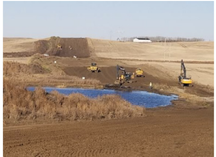
Wetland ramp removal – SF 42 - Oct 21, 2018
