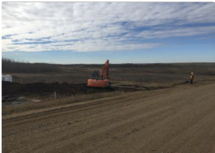
Excavator/dozer working on access – SF 43 - Oct 16, 2018
