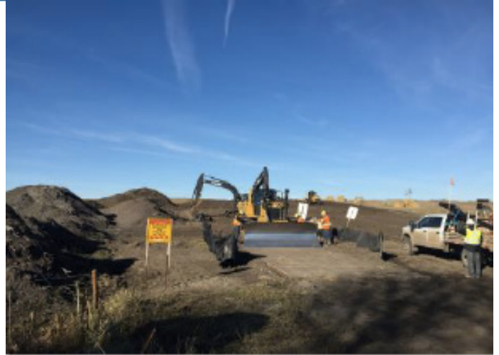
Utility crew cleaning dozer – SF 30 - Oct 19, 2018
