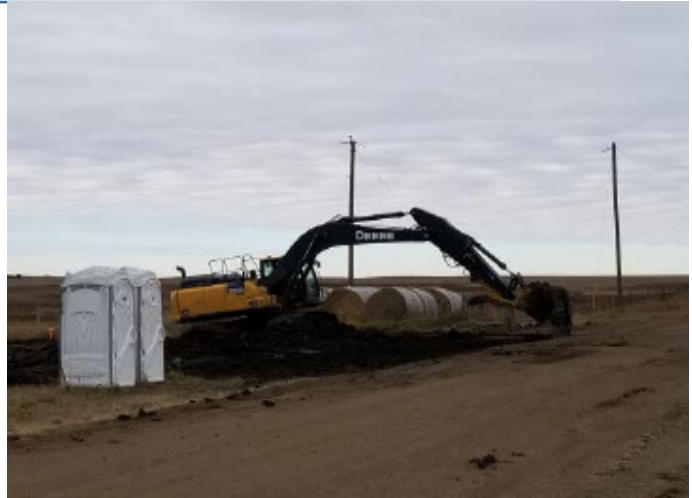
ROW ramp removal – SF 39 – Oct 16, 2018
