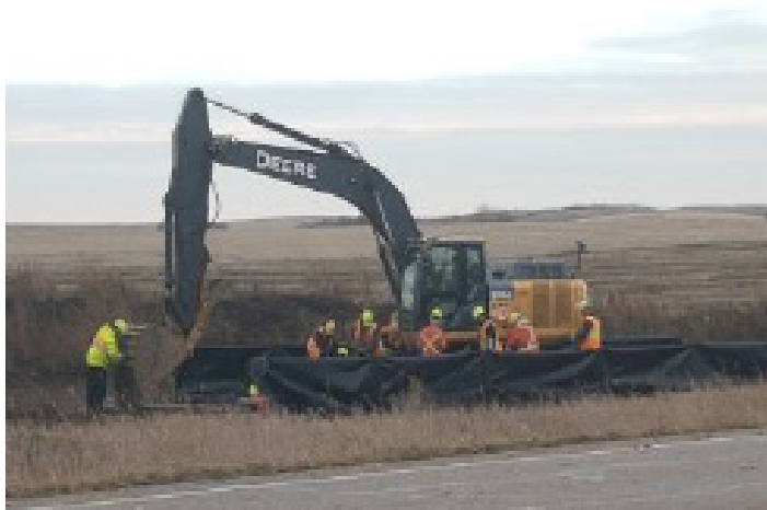
Crews cleaning excavator – SF 25 – Oct 16, 2018
