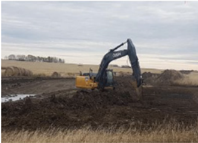
Excavator working on subsoil – SF 27– Oct 15, 2018
