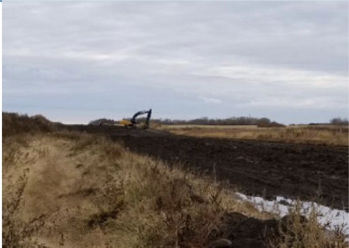
Excavator drying out subsoil - SF 57 – Oct 16, 2018
