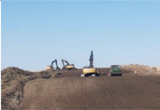
Decompacting and spreading out seconds - SF 49 - Oct 21, 2018
