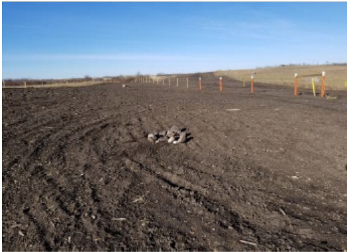
Rock piling on ROW - SF 21 - Oct 19, 2018
